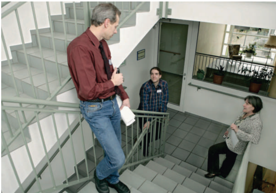
44 Staircases: adequate surfaces in good condition, continuous handrails and optimum lighting are prerequisites for preventing slip and trip accidents.
